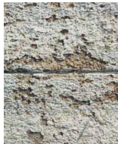
White rust on a galvanized steel tower basin. The reddish brown color is evidence of corrosion to the steel substrate.
